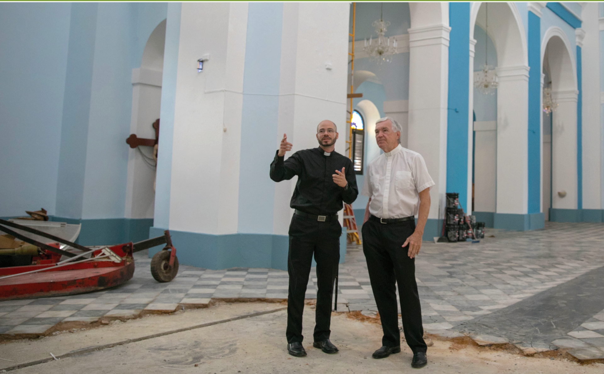
Father Jorge Morales, pastor of Our Lady of the Rosary parish in Vega Baja, Puerto Rico, shows Father Wall the hurricane damage to his historic church.
