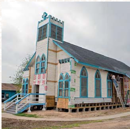
Renovation of Immaculate Conception Church in Lopezeville, Texas in 2013
